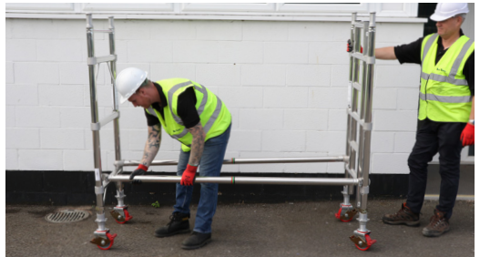
4. Fit 2 horizontal braces to the vertical member of the frames above first rung. Horizontal braces fit on from the inside of the tower facing outwards. (Integral ladder must be on the right hand side)
