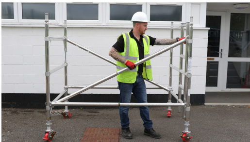
5. Fit 2 diagonal braces from the 1st rung to the 3rd rung in an alternate pattern.
